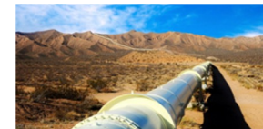
Oil pipeline monitoring
